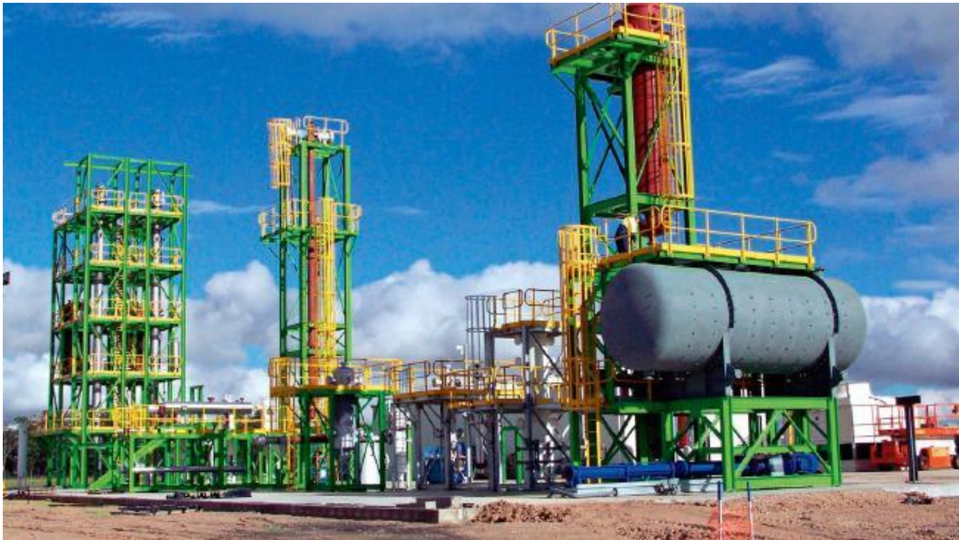
Linc Energy's underground coal gasification pilot plant at Chinchilla.
